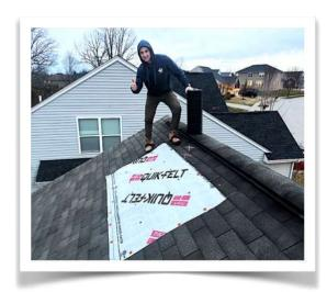
First, let's consider Synthetic Felt Installation for blocking off smaller areas. The advantage of this technique is that you don't need to overlap the ridge, limiting the area that you will have to damage with cap nails.
