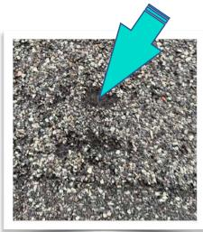
Blistered asphalt shingles may not always be a reason for a roof leak but they make the roof more susceptible to leaks.
