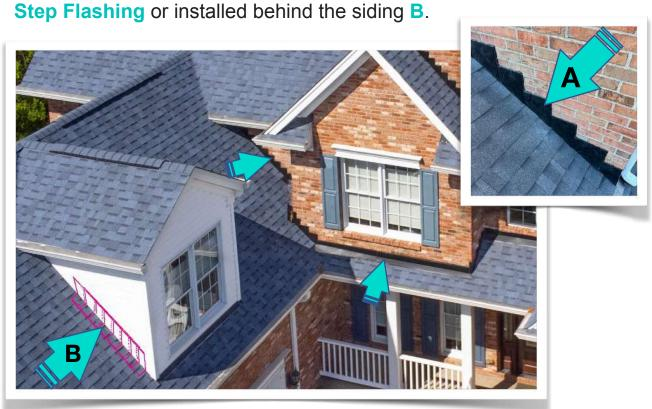
Often the leak comes from damaged or improperly installed flashing.
