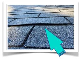
Popped nails do not lay flat to the roof, thus lifting the shingles, leading to a leak.
