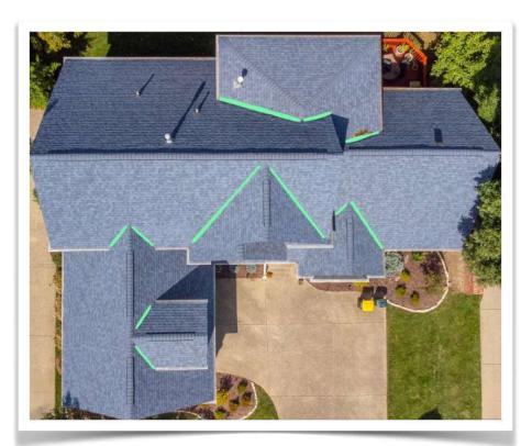
A roof valley is formed where two roof slopes meet.
