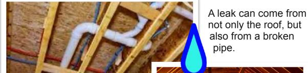
For this reason, if you find wet insulation in the attic, but do not see an obvious roof leak, check the HVAC pipes, water heater pipes, and any other water system pipes in the attic space!
