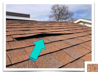
A nail usually pops up when the temperature changes. Expansion and contraction can cause the nails to pop up and lift the shingles. Improving the ventilation of your attic space will decrease the chances of that happening.
