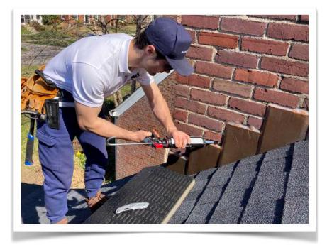
Silicon or caulk alone might not be a good enough solution to keep water away from flashing that is installed at the base of the chimney without a chimney cap.
