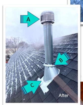
A leak usually occurs if the crown cap **A**, the middle cap **B**, or the flashing **C** are not installed/missing (see picture), or ice guard has not been installed around the base of the HVAC pipe.
