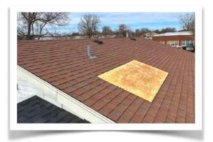
In the cases where the roof has a large hole created by something like a fallen branch, cover it with a 1/2-inch or thicker sheet of plywood or OSB. Use screws to secure it in place.
