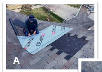
Even in the case of larger damage, if the affected area is not near a valley, two pieces of felt can be overlapped (just like giant shingles) starting at the the lower side of the slope.
