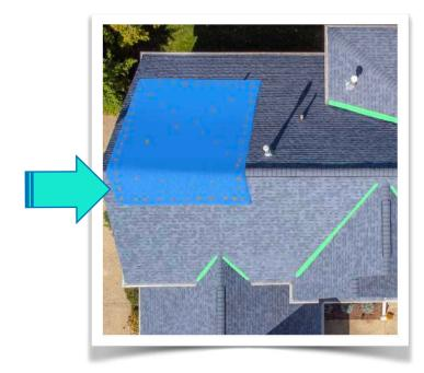
Tarp installation is a bit different. The tarp edges are folded and thicker. It is very hard to tuck them under shingles. This is why tarp is usually installed by **overlapping the ridge** to prevent water from entering under the tarp.
