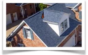
When the leak source in the valley is close to the ridge, it is easier to cover it with a tarp.
