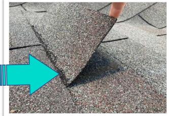
This is what makes shingles vulnerable to wind damage. The wind can flip the loose shingle tabs, gradually loosening the nails that secure them. You will usually notice a crease on the shingle tabs that are no longer adhering.
