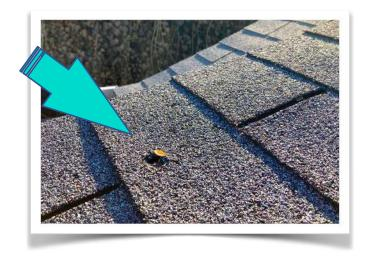
•If the pop nail penetrates the shingle, like in this example, the nail can be removed and the hole sealed with silicon or roof caulk. But be careful! Too much could compromise your insurance claim, so consult a professional if you are not sure.
