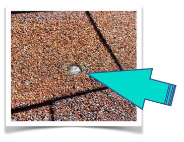
Improperly installed shingles can block trapped moisture. If the adhesive wasn't applied properly, moisture can accumulate and evaporate under your shingles. During hot days this trapped moisture expands, sometimes along with vapors from the heated asphalt layer, resulting in **blisters**.
